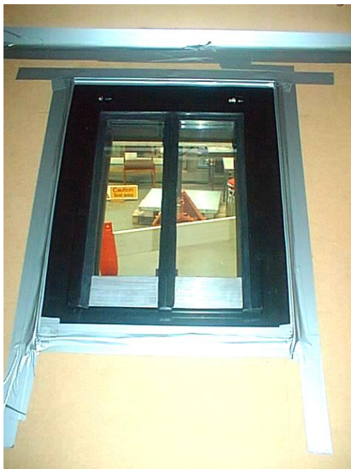
Figure A4. The outdoor face of the specimen roof light
